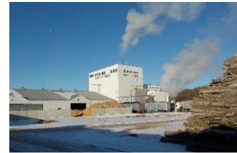
Kobe Bussan's Woody Biomass Power Plant
